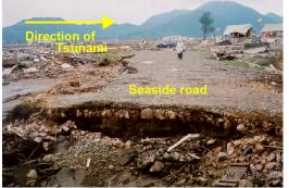
Fig. 1 : Erosion of seaside road due to tsunami (Indonesia)
