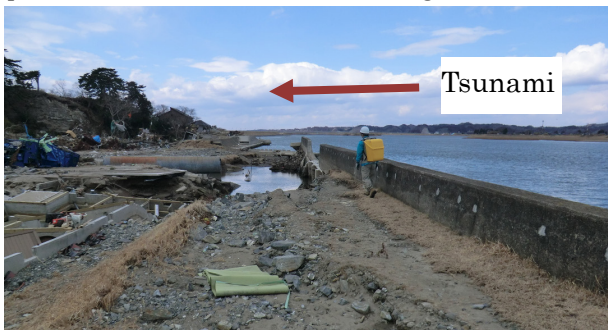
Fig. 1 : Erosion at backside du to tsunami (2011 Great Eastern Japan Earthquake Tsunami)
