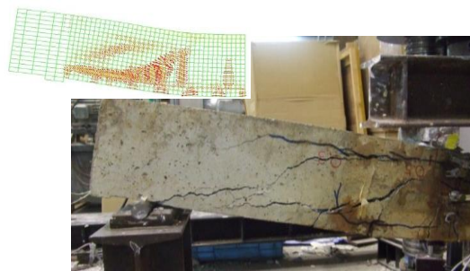
Fig.3 Flexural loading test and FE analysis result of RC beam with the corroded reinforcements
