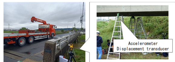
Check the health condition of the structure by vibration characteristics
