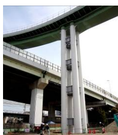
New type of steel pier with steel pipes
