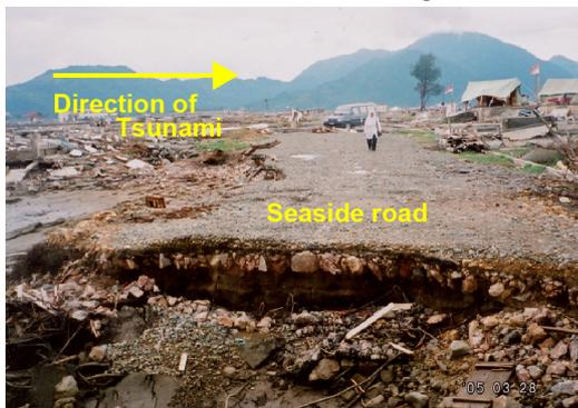
Fig. 1 : Erosion of seaside road due to tsunami (Indonesia)
